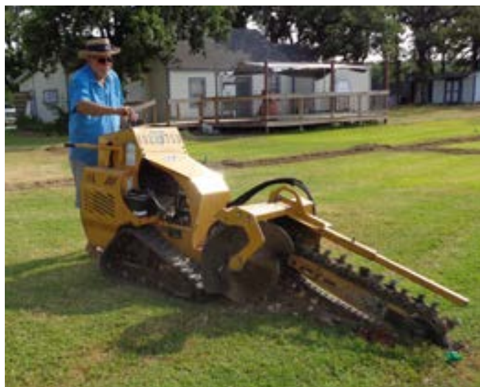
Trenchmaster Dave makes the dirt fly.
